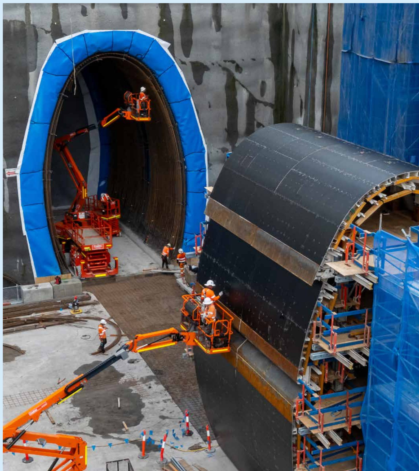
Tunnel nozzle excavation at Sydney Olympic Park Metro Station site.
