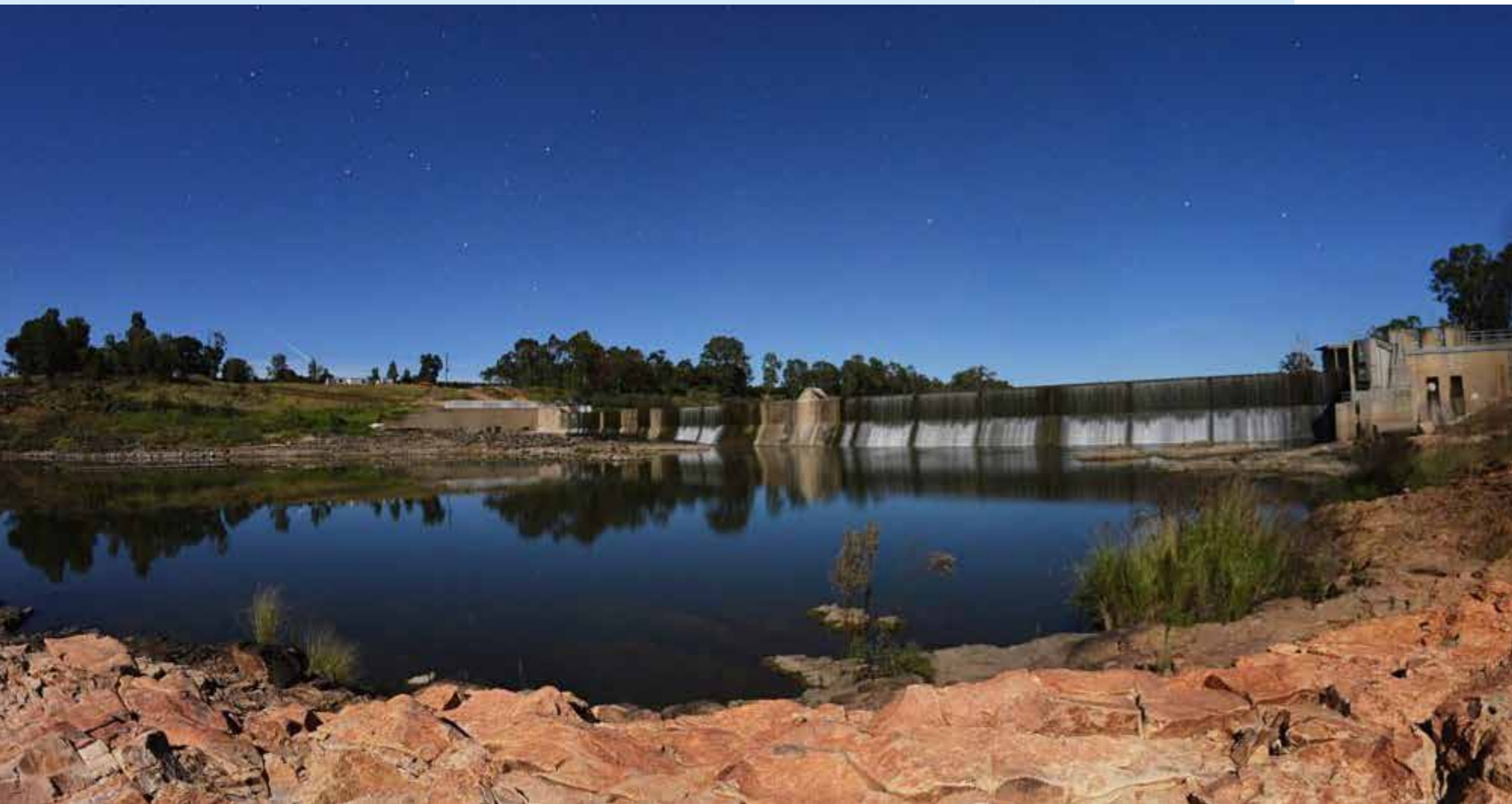
Figure 5 Gonyah water supply infrastructure, QLD (9)
