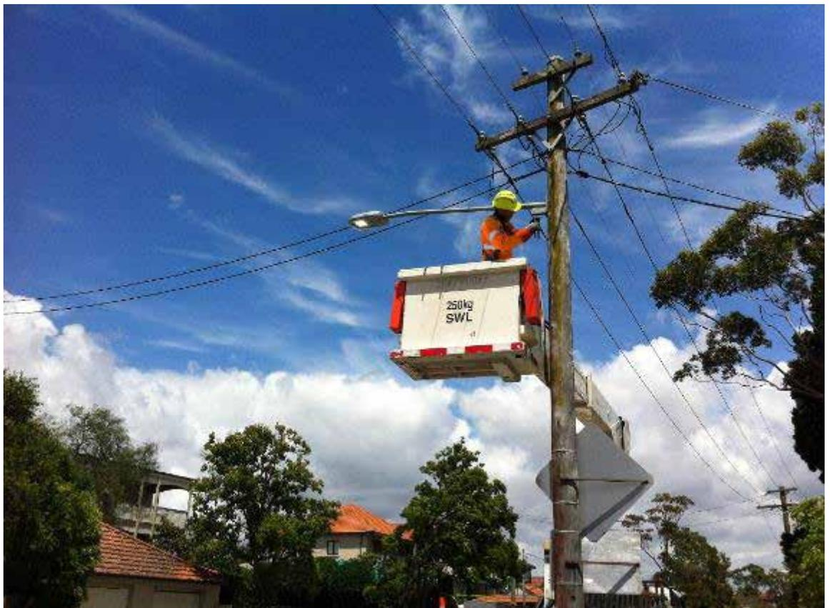
Replacing outdated technology with new efficient LEDs. Image: Ausgrid
