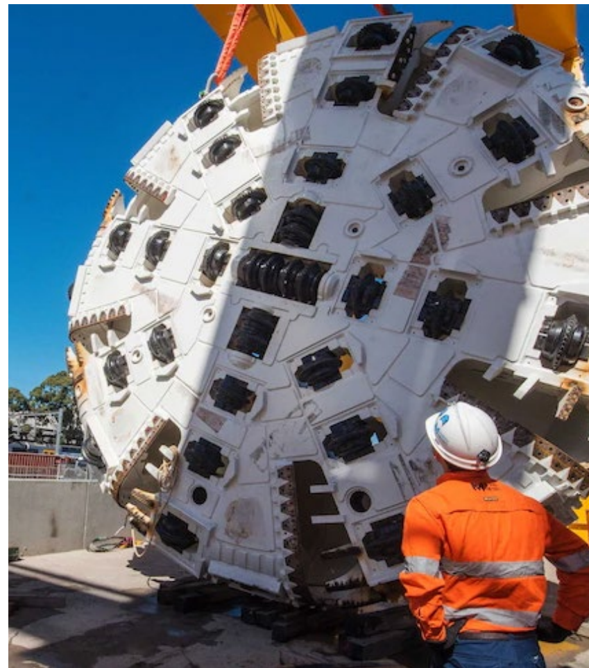
NSW's tunnel boring machine in use on Metro rail construction.
